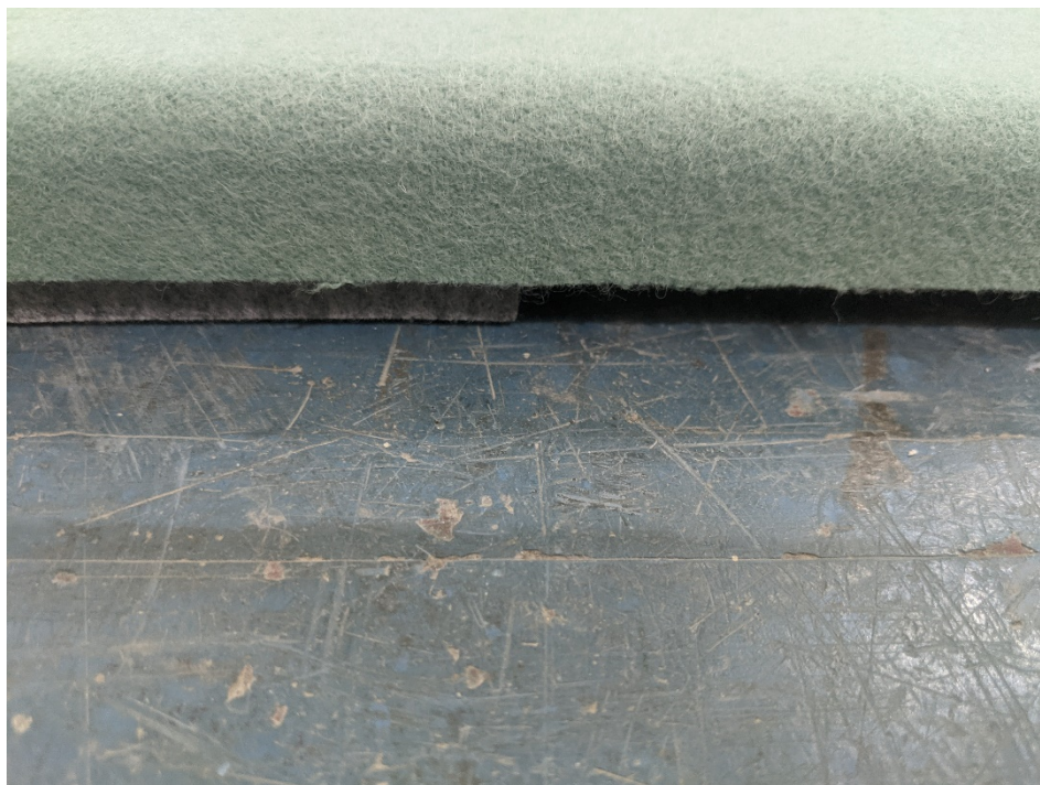
Figure 4 – Air space resulting from felt mounting brackets
